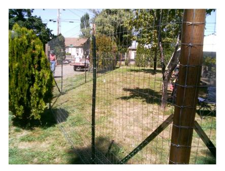
**STEP 6 – Stretch your fence:** When concrete is set, attach the welded wire fencing. Begin by standing the rolled fence upright along the perimeter of the enclosure. Line up one end of the fencing and use fence staples to secure it to the post (as shown in photo). Roll the fencing along the perimeter to the next corner post and attach the fence-stretcher. Use the come-along to stretch the fence until it is taut, having helpers on hand to make sure the fencing doesn't
